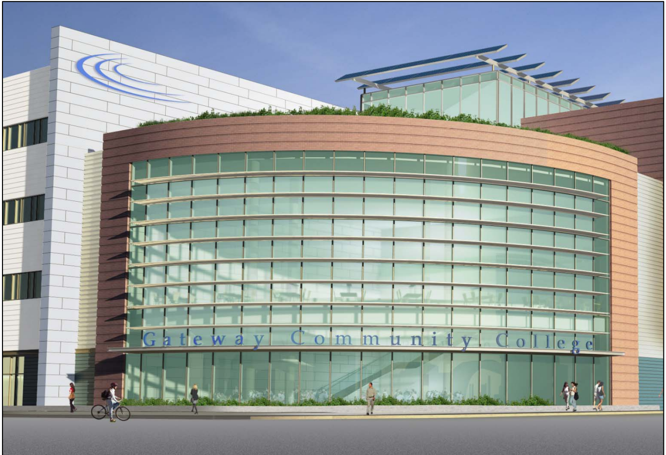
AI.8: Exterior View Looking North
